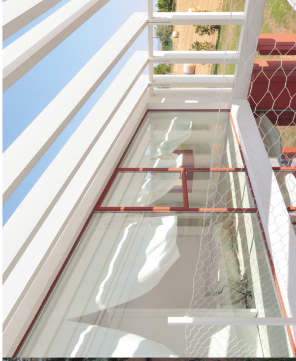
Single-leaf window with consistent joints around the entire perimeter, including the fixed bottom section.
