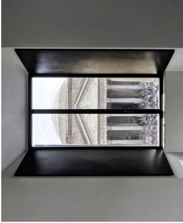
Double casement window with 47 mm sections constant around the perimeter and a central mullion of 62 mm.
