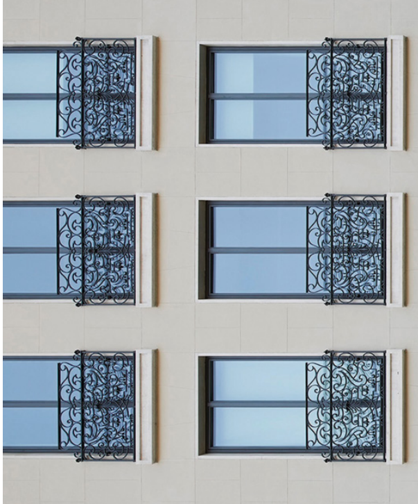
Double casement windows with constant 62 mm sections, both around the perimeter and in the central mullion.
