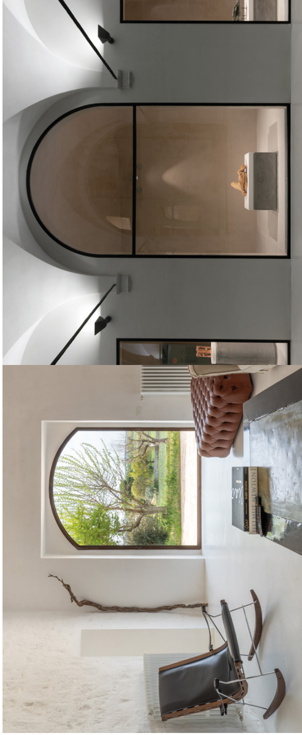
Vertical pivot window frame with constant sections around the perimeter and concealed hinges.
